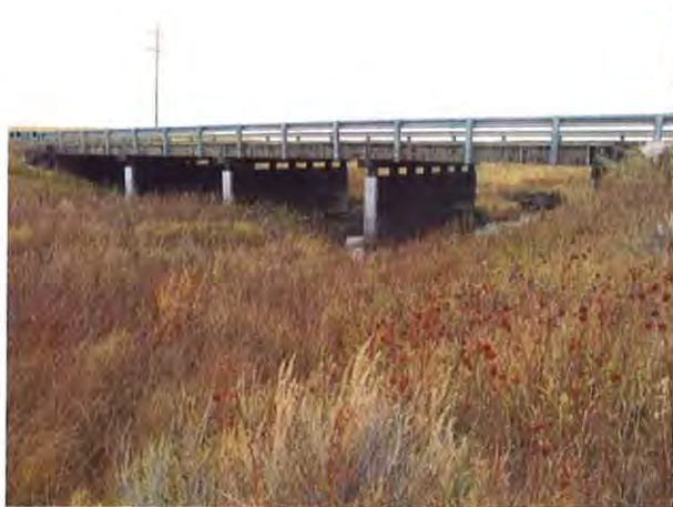
Bridge at Hwy 66 Crossing
